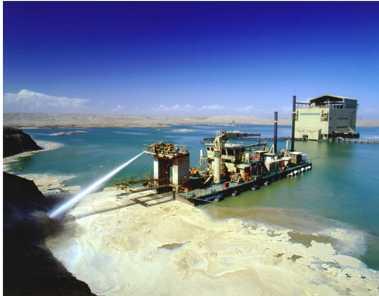
Figure 1: Beachcomer Dredge and Floating Treatment Plant
