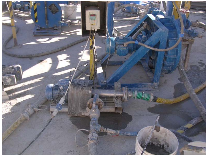
Figure 2 Shear device installation
